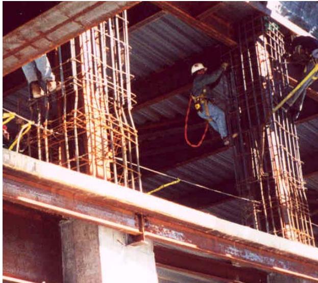
Figure 1- Composite column in which steel section is used mainly for carrying construction loads (low reinforcement ratio).
