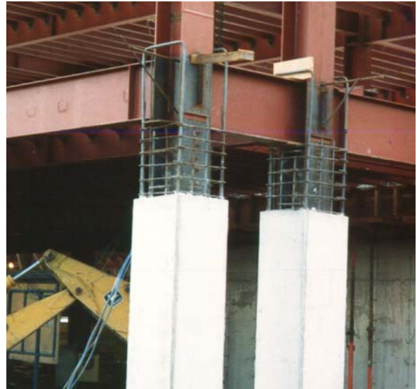
Figure 2- Composite column in which steel section provides most of the strength and stiffness (high reinforcement ratio).
